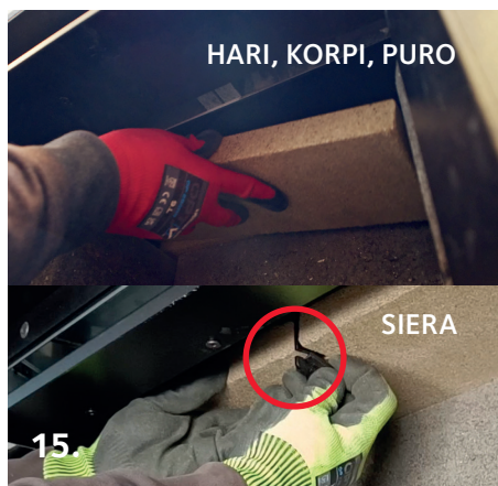
Remove the baffle plate at the front and the clean-out from the upper part of the firebox. Note! Siera is equipped with a locking clip that must be opened. Sweep out the front and rear ducts of the fireplace through the clean-out.
