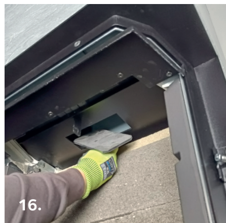
Remove the baffle plate at the front and the clean-out from the upper part of the firebox. Note! Siera is equipped with a locking clip that must be opened. Sweep out the front and rear ducts of the fireplace through the clean-out.
