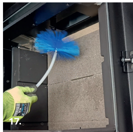
Remove the baffle plate at the front and the clean-out from the upper part of the firebox. Note! Siera is equipped with a locking clip that must be opened. Sweep out the front and rear ducts of the fireplace through the clean-out.
